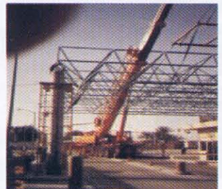
Space frame for Saudi Aramco Station #4
