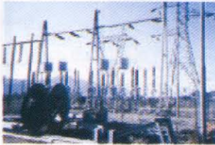
Sub-station yard equipment installation for SCECO-South
