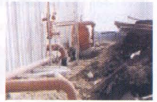
Fire protection works
