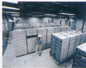
Batteries for UPS of Expec computer center (S. Aramco)
