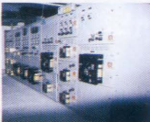
LV switchgear serving Expec computer center (Saudi Aramco)
