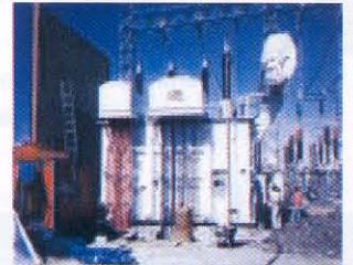
Installation of 133 & 70 MVA transformers
