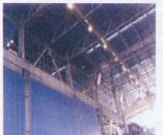
Haded flat product facilities (Electro-Mechanical works)
