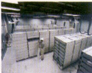
Batteries for UPS of Expec computer center (S. Aramco)
