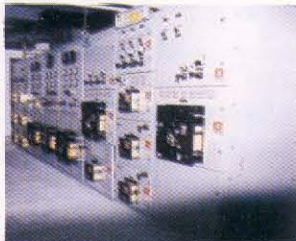
LV switchgear serving Expec computer center(Saudi Aramco)
