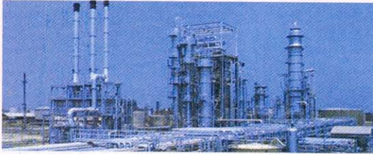
Mechanical & Electrical Construction
