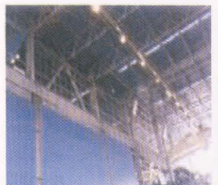
Hadeed flat product facilities(Electro-Mechanical works)
