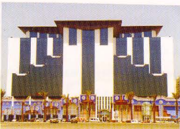
Mahmood Saeed Plaza - Jeddah HVAC Works Completed in Aug-1999
