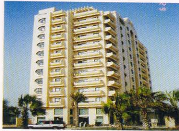
Al Nauras Tower - Jeddah Electro-mechanical Works Completed in April-1997
