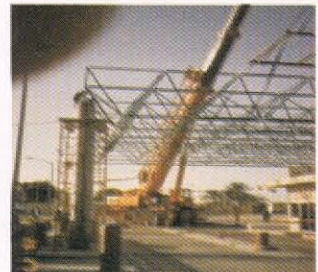
Space frame for Saudi Aramco Station #4
