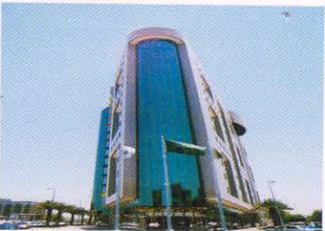
Saudi Business Centre - Jeddah HVAC Works Completed in May-1999
