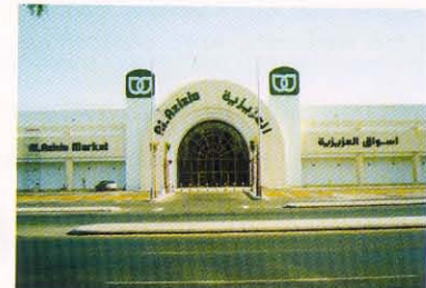
Al Azizia Market - Jeddah Electro-mechanical Works Completed in May-2001
