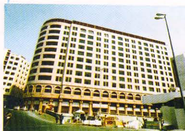
MAKKAH Sofitel HVAC Works Completed in Nov-2001
