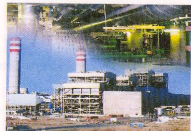
Shoaiba Steam Power Plant HVAC Works Completed in June-2002
