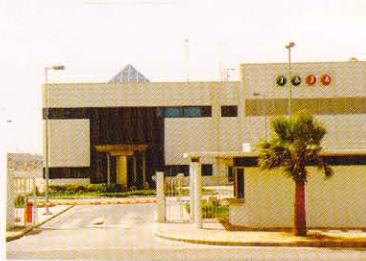
SAJAPHCO - Jeddah HVAC Works Completed in May-1999
