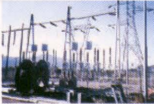
Sub-station yard equipment installation for SCECO-South
