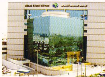
Al Bank Al Saudi Al Fransi - Jeddah Electro-mechanical Works Completed in June-2000
