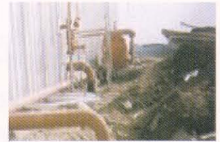
Fire protection works
