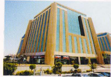
Jeddah Businessmen Centre HVAC & Electrical Works Completed in Feb-1998
