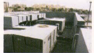
HVAC units serving Low Voltage switchgear building (Saudi Aramco)
