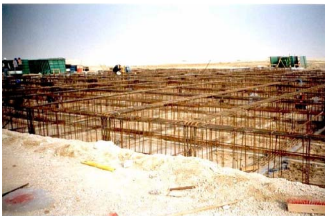
Plate 1: Excavation & Rebar Placing For Stiffened Slab Waffle Foundation at the Site
