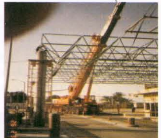
Space frame for Saudi Aramco Station #4
