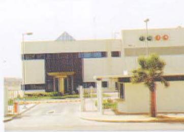
SAJAPHCO - Jeddah HVAC Works Completed in May-1999
