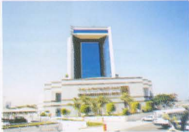
Jeddah Chamber of Commerce Electro-mechanical Works Completed in March-1991
