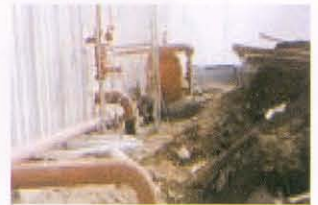
Fire protection works
