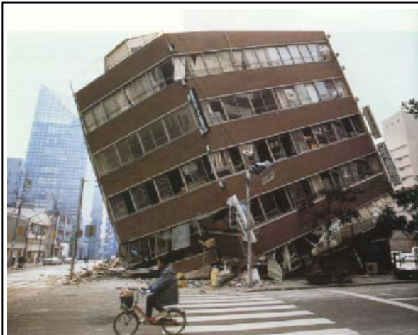
Figure 8: A Building after Earthquake, Kob
