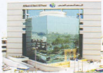
Al Bank Al Saudi Al Fransi - Jeddah Electro-mechanical Works Completed in June-2000
