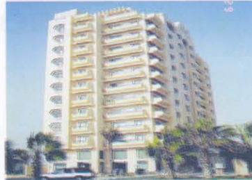
Al Nauras Tower - Jeddah Electro-mechanical Works Completed in April-1997
