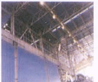
Hadeed flat product facilities (Electro-Mechanical works)
