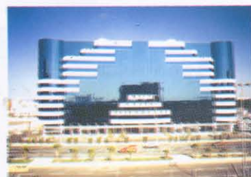
Farsi Centre - Jeddah Electro-mechanical Works Completed in June-2001
