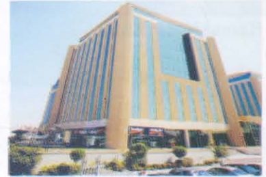
Jeddah Businessmen Centre HVAC & Electrical Works Completed in Feb-1998
