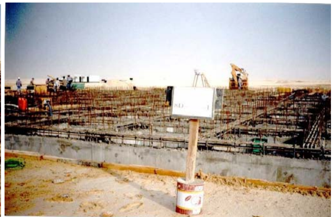
Plate 2: Concrete Placing In Stiffened Slab Waffle Foundation at the Site
