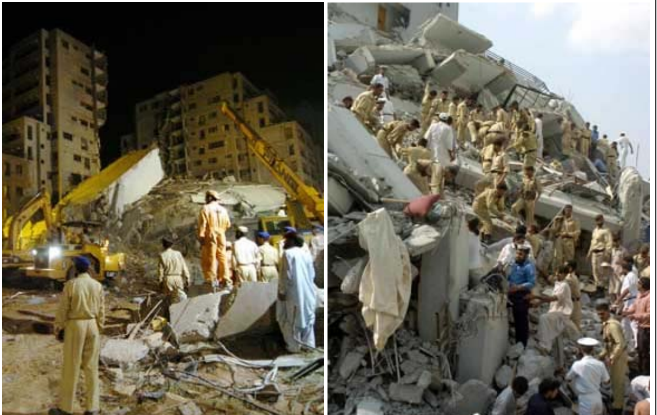
Figure 10: Rescue Operation at the Site of Toppled Margalla Tower in Islamabad
