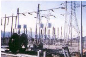
Sub-station yard equipment installation for SCECO-South
