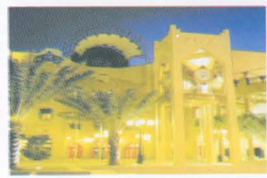
Al Tameer - Riyadh HVAC & TESS Works Completed in Aug-1999
