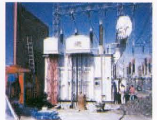
Installation of 133 & 70 MVA transformers
