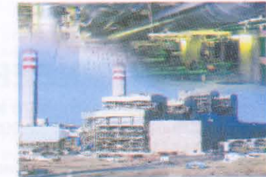
Shoaiba Steam Power Plant HVAC Works Completed in June-2002
