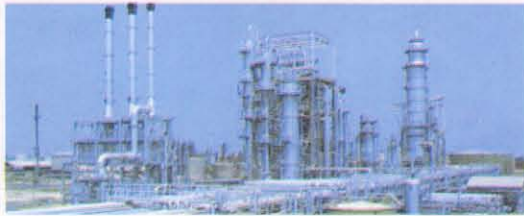
Mechanical & Electrical Construction
