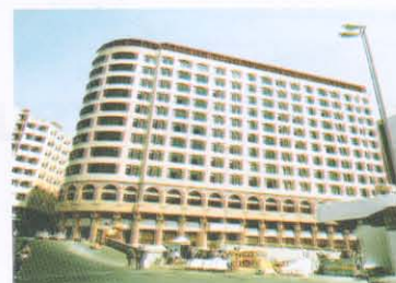
MAKKAH Sofitel HVAC Works Completed in Nov-2001
