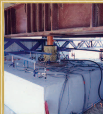
Stone Column Testing
