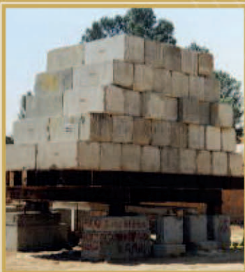
Pile Load Test
