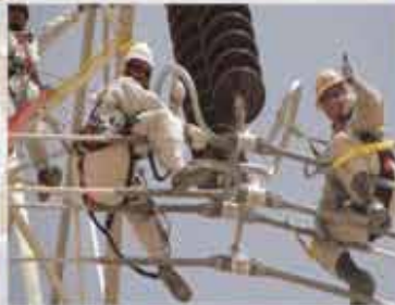
380kV Live Line Training
