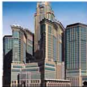
Residential and Commercial Building
