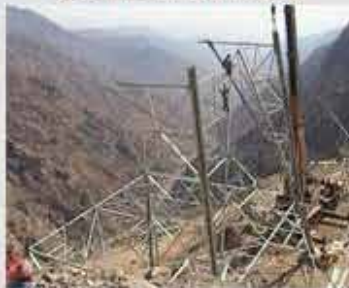
380 kV Makkah-Taif Tower Erection
