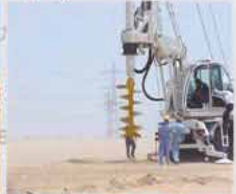
380kV Auger Foundation
