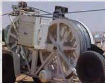
Pulling of 132kV Conductor
