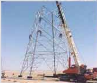
380kV Tower Erection
