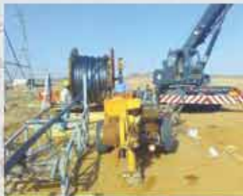
U/G Cable Pulling in Progress
