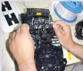
Splicing, Jointing of OPGW
