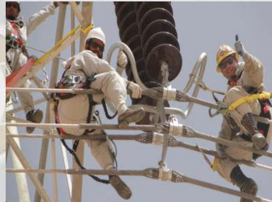
380kV Live Line Training
