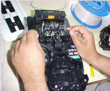
Splicing-Jointing of OPGW
