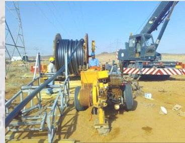
U/G Cable Pulling in Progress
