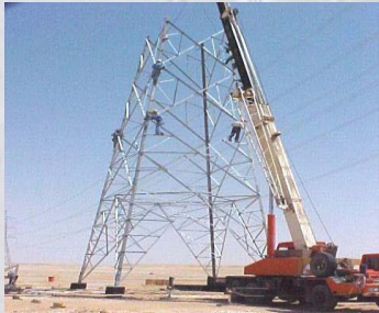
380kV Tower Erection
