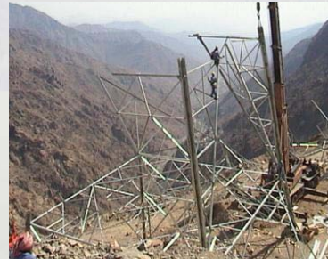
380 kV Makkah-Taif Tower Erection
