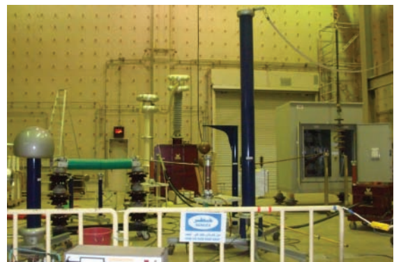
Figure 1: Test setup for impulse and power frequency voltage tests on switchgear panel
