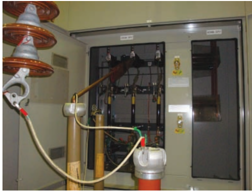
Figure 2: Test connection on switchgear panel
