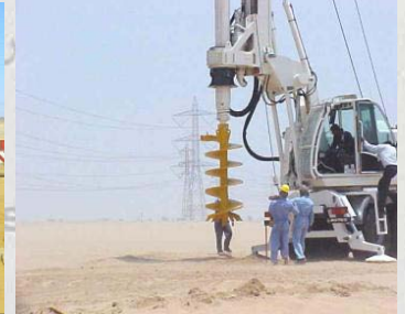
380kV Auger Foundation
