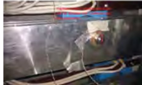
Figure 3 – Sensor installed on the LV busbar
