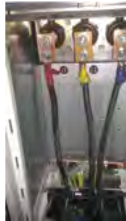
Figure – 4 Generator connections
