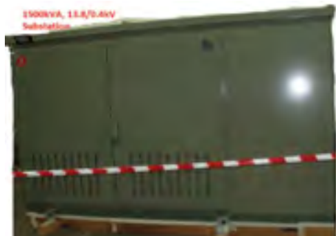
Figure 1 – Substation in the test room prepared for temperature rise test.
