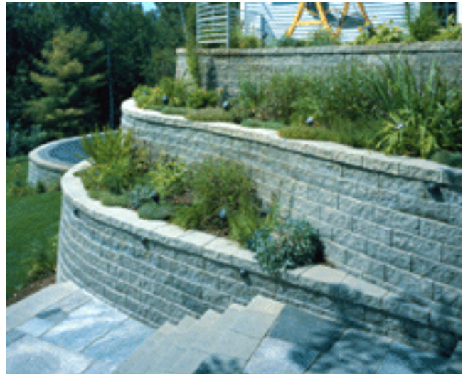
Plate-2: Landscaping in Front of a Villa
